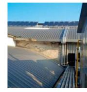
Photo 10. Solar collectors (62 m², 27 collectors)
