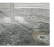
Photo 6 Sealed connections of accessories
