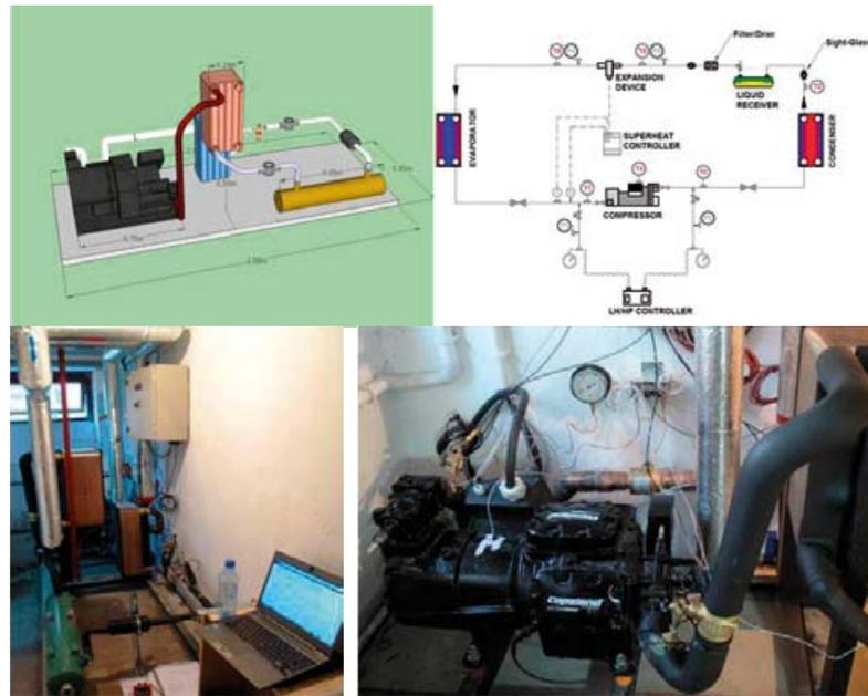
Figure 18. Schematic Sensor Positions and Images of the Heat Pump on site.
