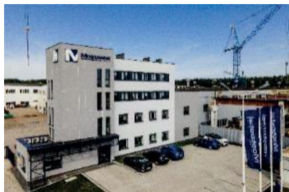
Mostostal Kielce S.A. Head office
