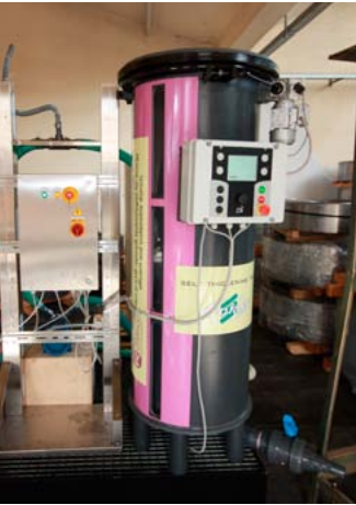
Food waste tank
