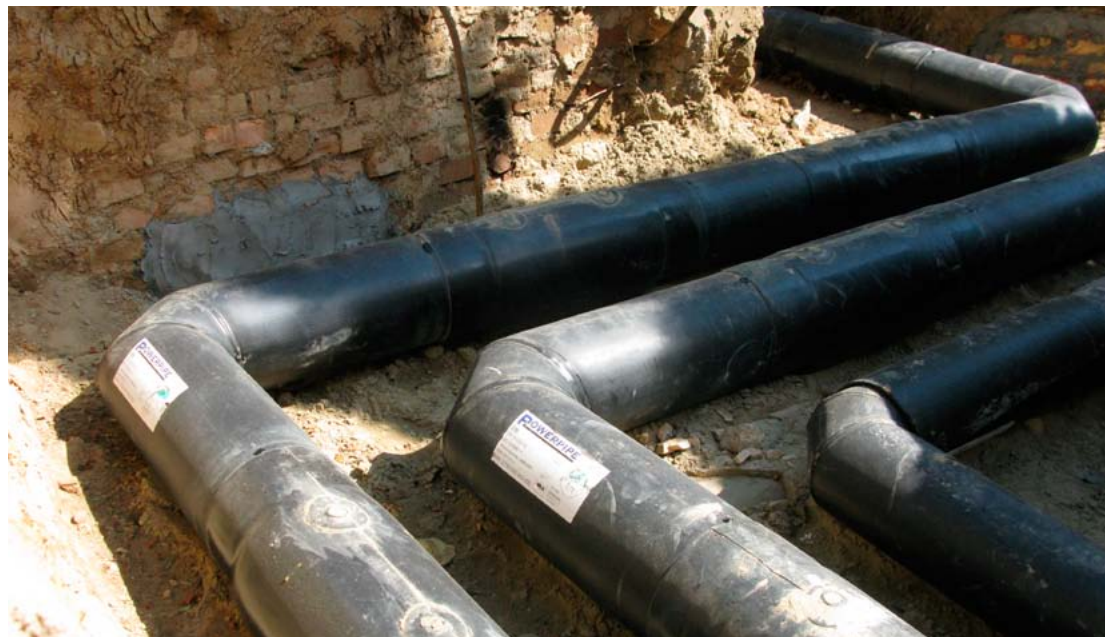
Hybrid insulated district heating pipes in excavation
