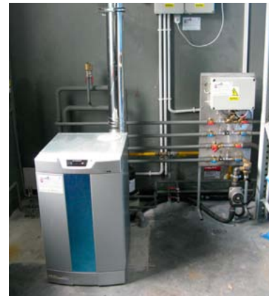
Stirling engine installed
