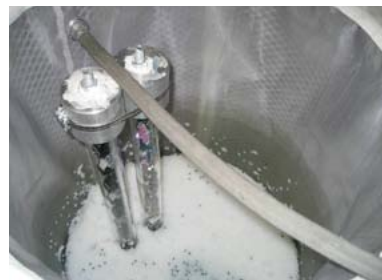
Level metering system
