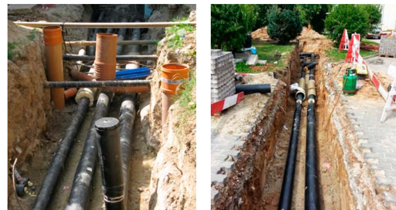
Building district heating network with use of prototype pipes
