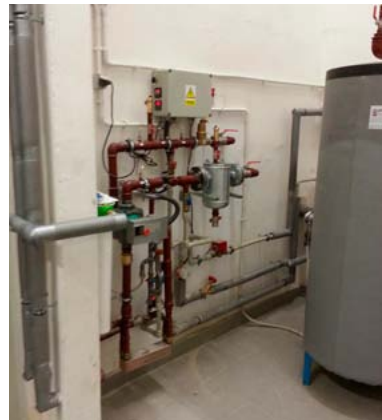
Main control room
