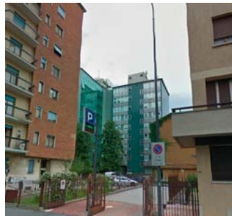
Demonstration building in Italy
