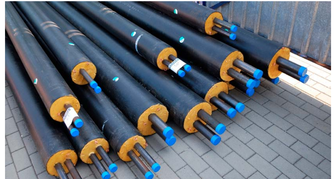
Hybrid insulated district heating pipes delivered to construction site
