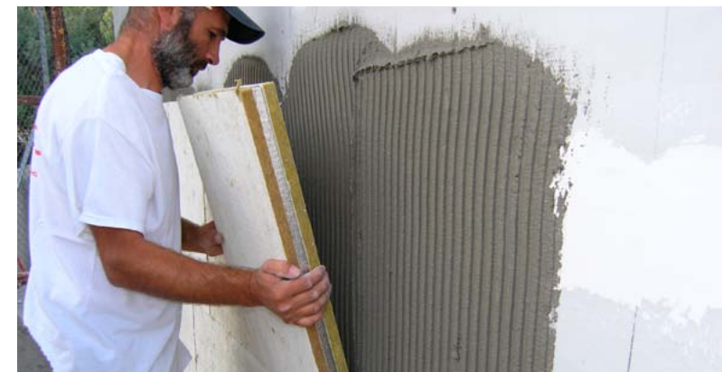
Installation of the new ETICS
