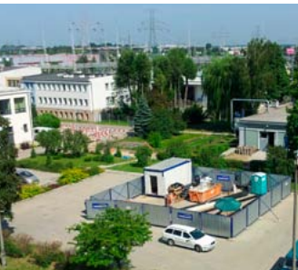
The pilot plant in Poland
