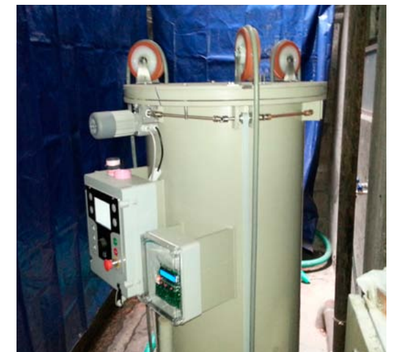
Food waste tank
