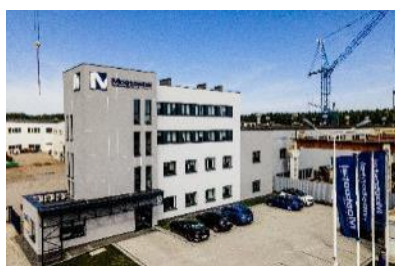
Headquarters of Mostostal Kielce S.A.
