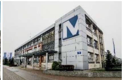
Head office of Mostostal Plock S.A.
